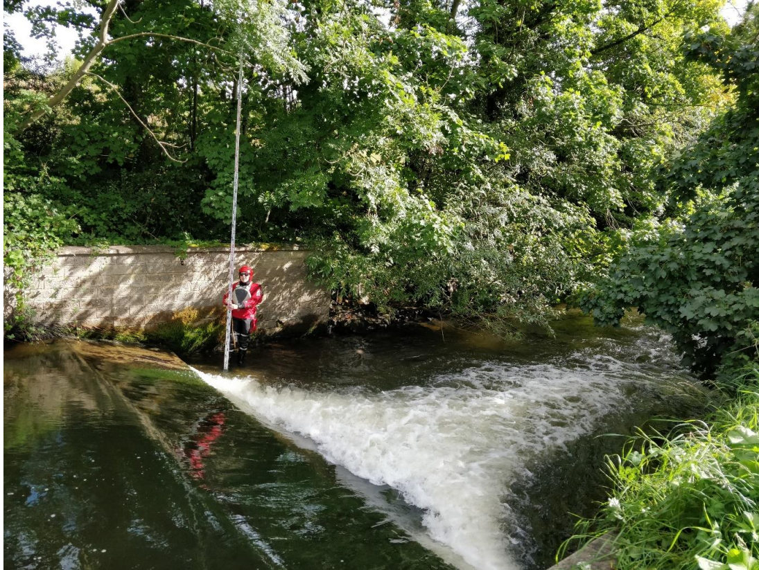
Figure 2.21 Tallanstown weir with one transversal: sloping weir face.
