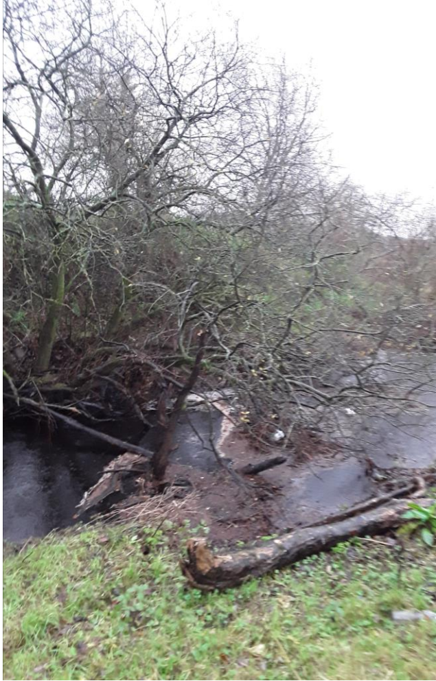
Figure 4.9 Photo of blockage in channel which will impede flood conveyance.
