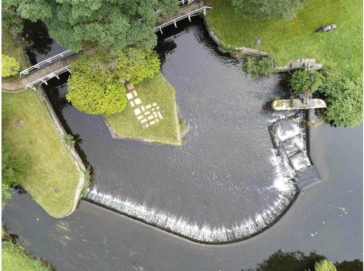
Figure 2.20 Castlebellingham weir has two transversals: fish pass and vertical weir face.
