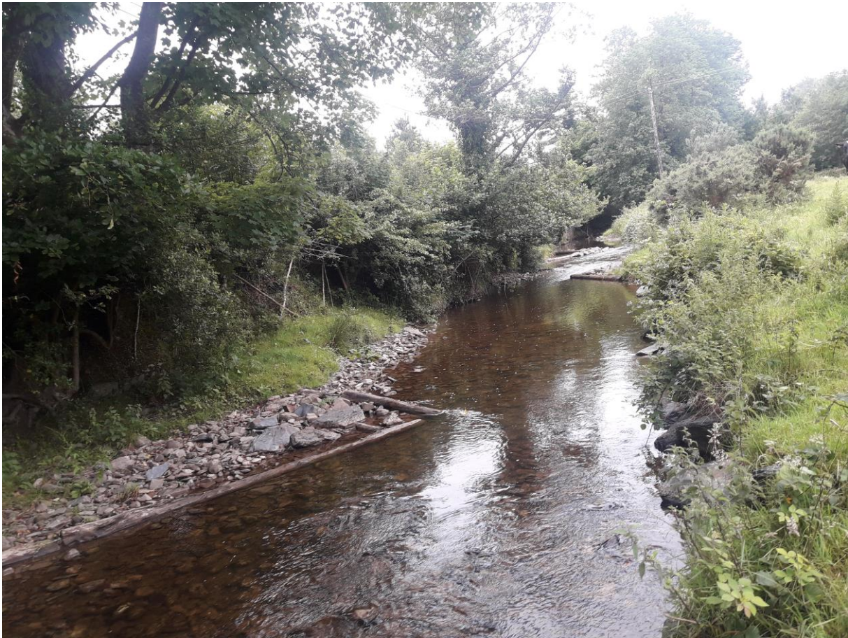
Figure 2.8 Deflectors on the Cormey River.
