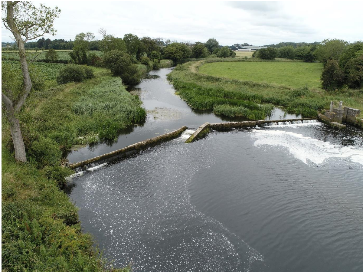
Figure 2.19 Lynns weir has two transversals: fish pass and sluice.
