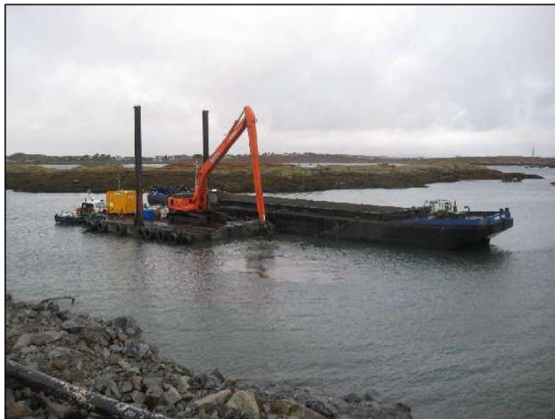
Figure 1 Typical Dredge Barge, Backhoe Excavator, and Hopper Barge
