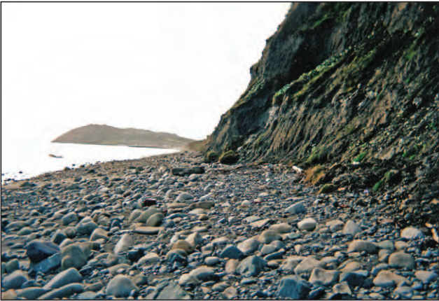
Plate 12.8 - View Southwards from immediately below Landfall A showing cliff erosion
