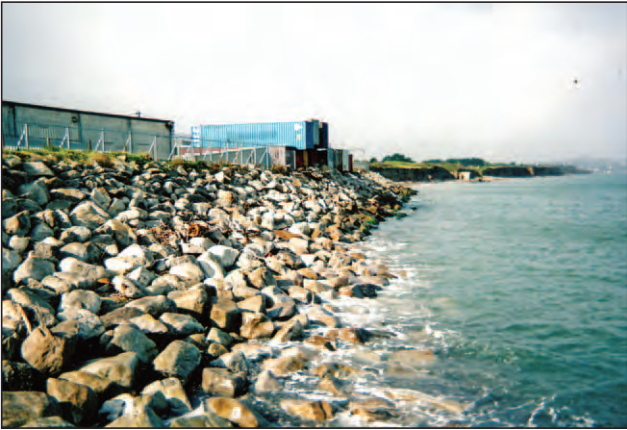
Plate 12.1 - Wave break protecting the compound looking north towards Landfall B
