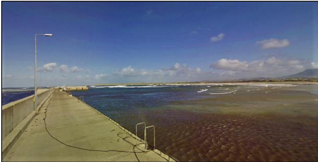
Photograph 2: Magheraroarty Pier (site for dredging)
