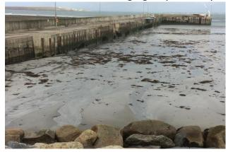
The photo to the left shows the typical state of Magheraroarty pier following winter storms with access only to the outer reaches of the pier at low tide. Most of the pier is inaccessible due to the accumulation of sand over the winter months with dredging now required to provide access along the pier for the upcoming season.
