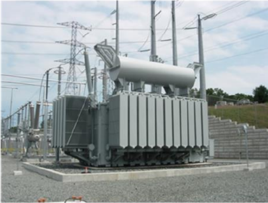
Figure 1: Typical shunt reactor for reactive power compensation [15]
