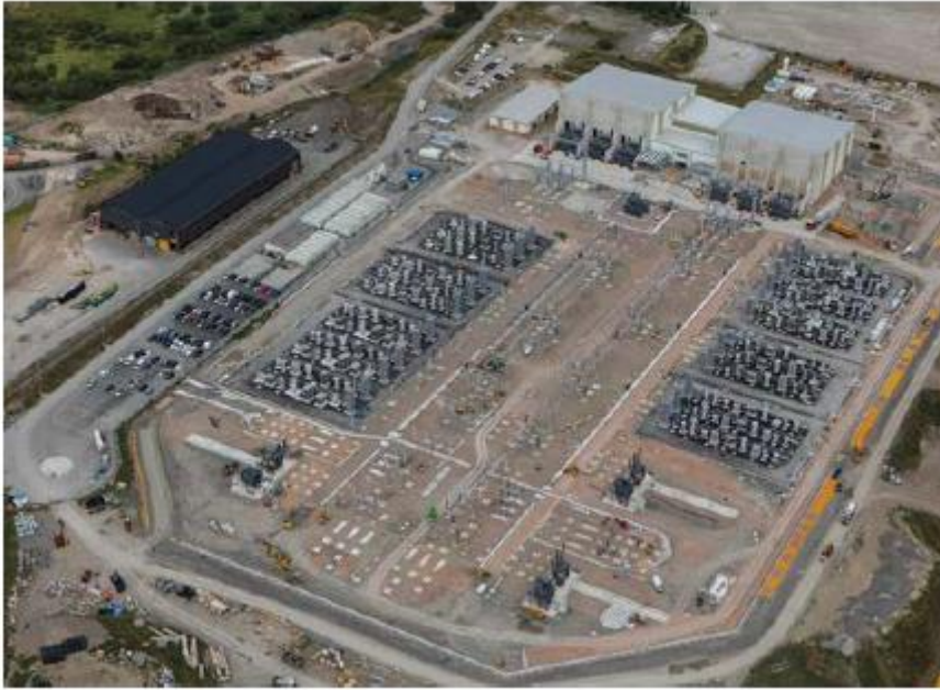
Figure 19: Aerial view of the converter station under construction at Hunterston [35]
