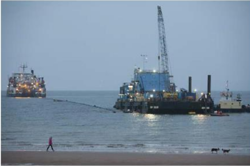
Figure 21: Cable laying vessel for the Western HVDC Link [36]
