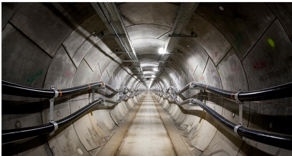
Figure 5: INELFE project: cables in tunnel section [28]
