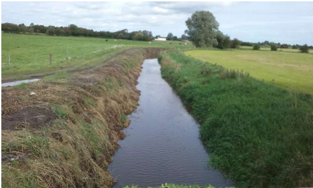
Figure 5.18 Site 10 – upstream view from Newbridge following maintenance in 2016. Evidence of low berm on left bank
