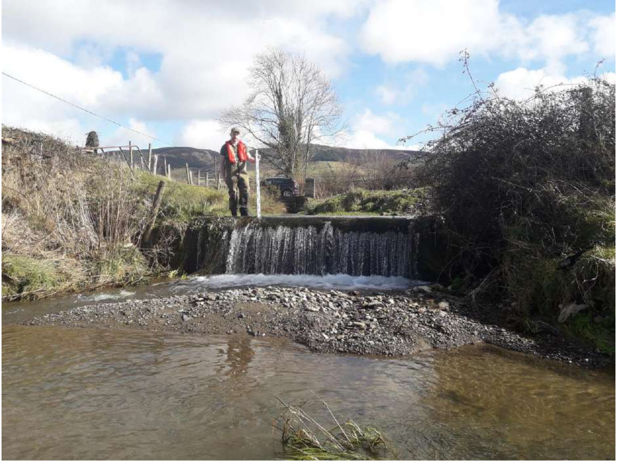
Figure 7.6 Gravel trap on the Ollatrim River, Nenagh Catchment (ST13).
