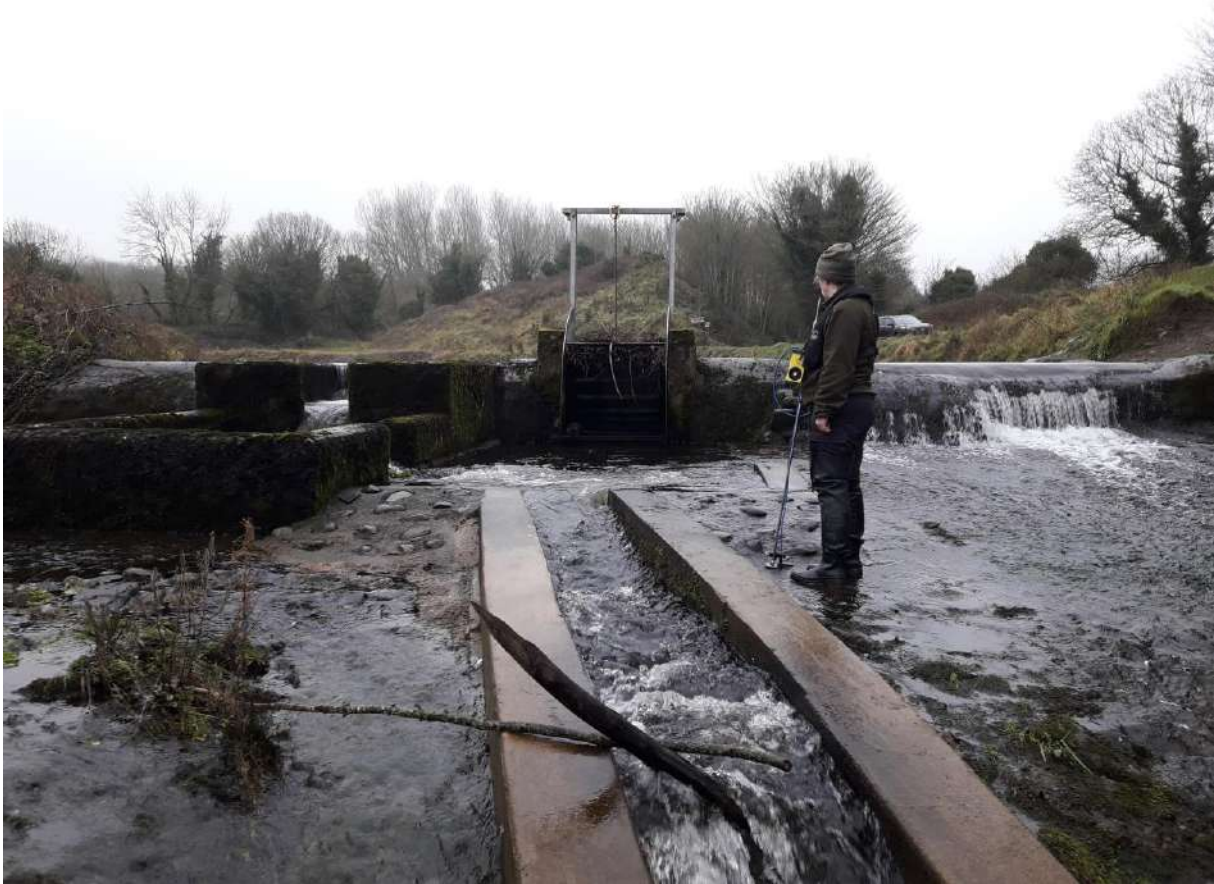
Figure 7.4 Gravel trap on the Kilcormac Silver, Brosna catchment (ST6).
