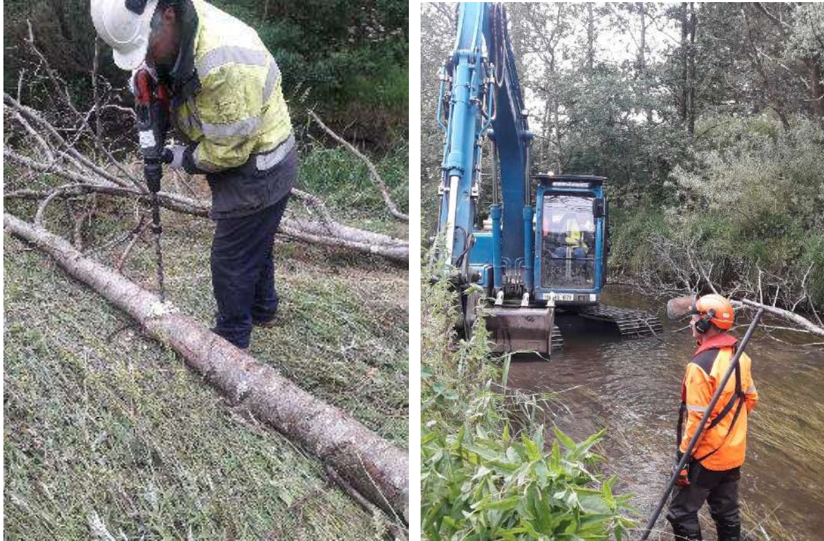
Figure 6.3 Photos of the various steps required to install the timbers.
