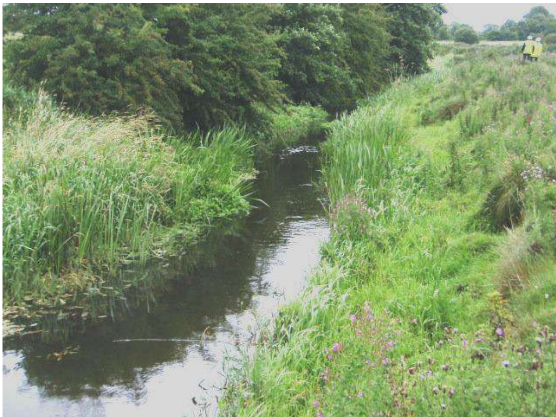
Figure 5.13 Tullamore Silver approx. 2007, showing open channel flow through a wedge-shaped cross section excavated in maintenance.
