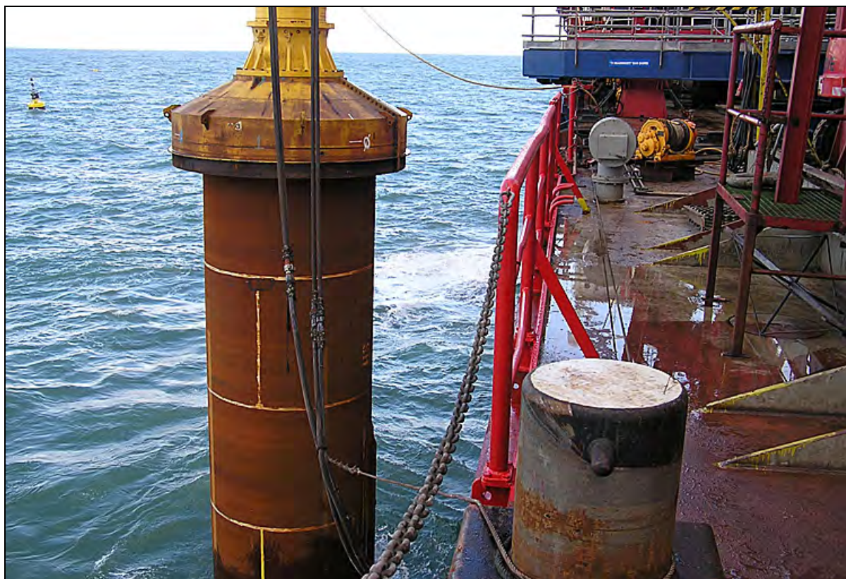
Figure 3.3 Installation of a steel monopile
