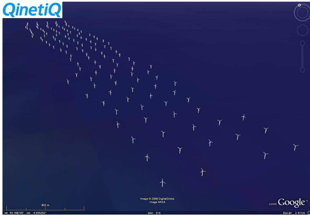
Figure 1 Kish and Bray wind farm plotted in Google Earth
