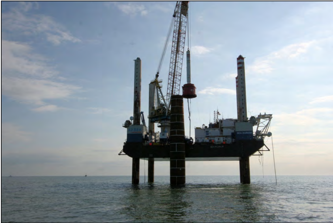
Figure 4.2 Installation of Steel Monopile at London Array Offshore Wind Farm
