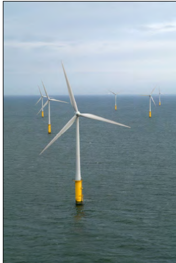
Figure 4.1 Typical Offshore Wind Farm (Photo courtesy Vestas Wind Systems A/S)
