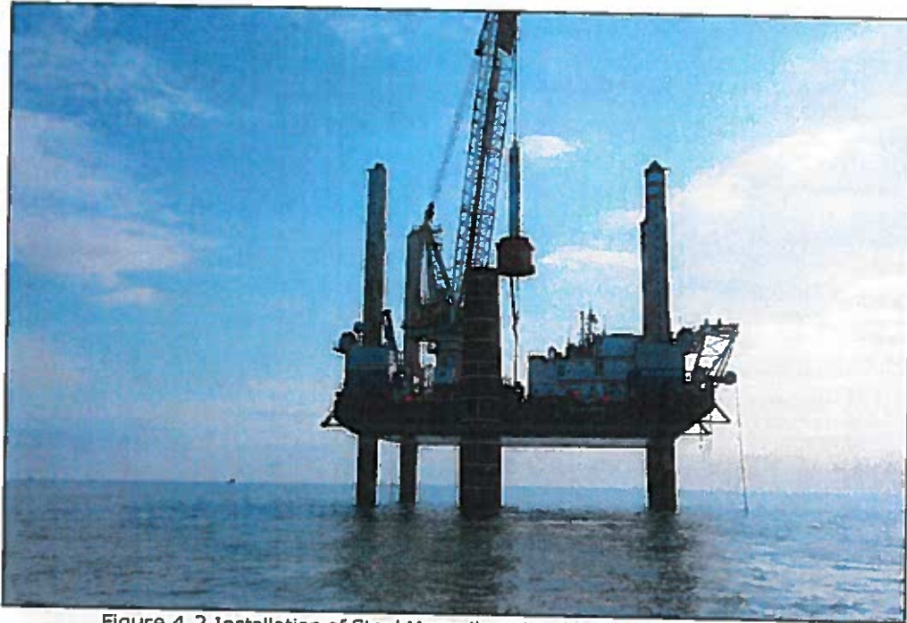
Figure 4.2 Installation of Steel Monopile at London Array Offshore Wind Farm
