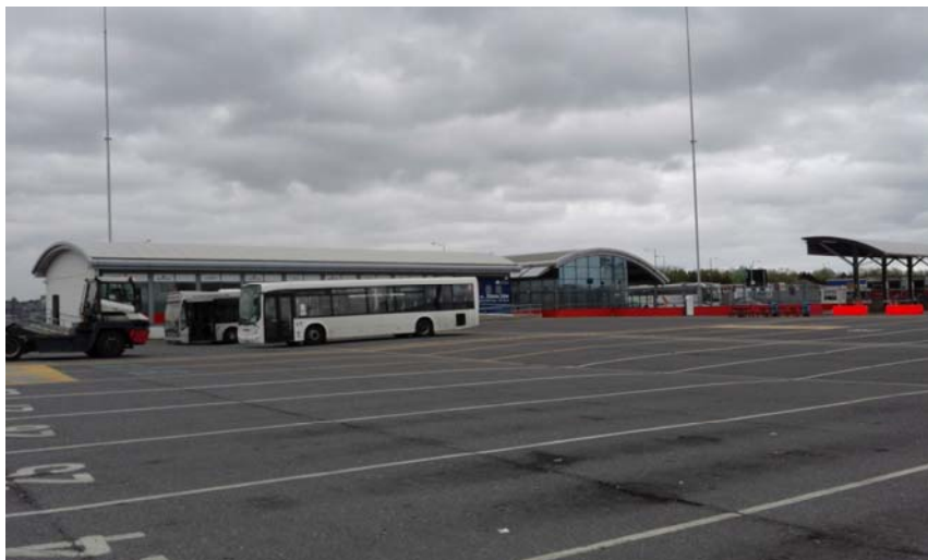
Plate 9: Existing Stenaline terminal
