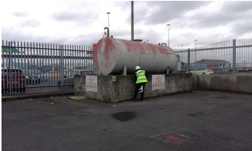
Plate 11: Fuel tank present directly west of Irish Ferries terminal building
