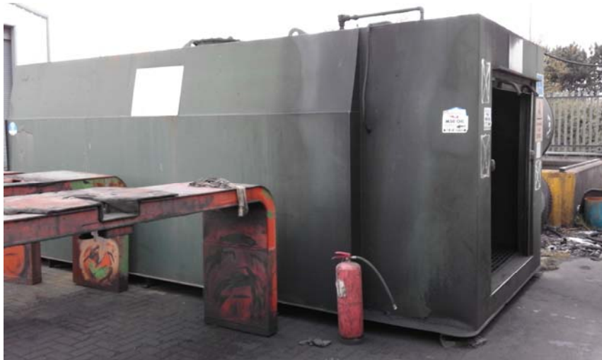
Plate 6: Fuel tank present in north of Zone A (Figure 3)
