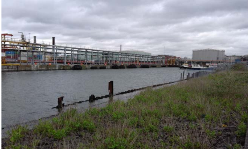
Plate 1: Area east of Oil Berth 4 to be infilled
