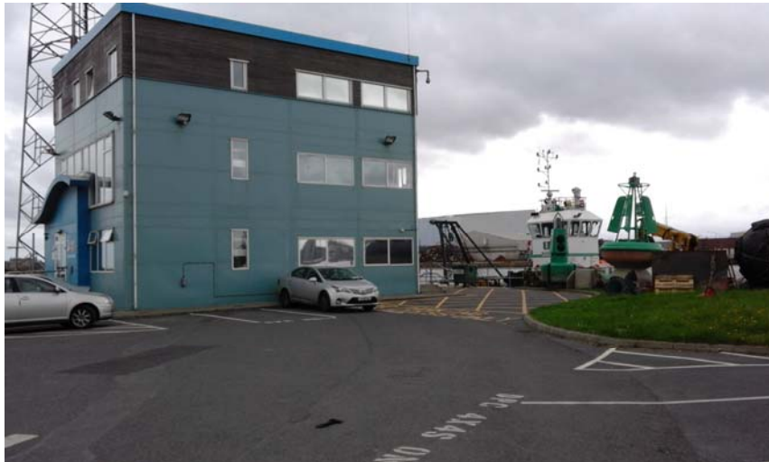
Plate 2: Dublin Port VTS building at the end of the old eastern breakwater (to be demolished)
