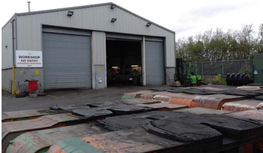
Plate 5: Garage area present in north of Zone A (Figure 3)
