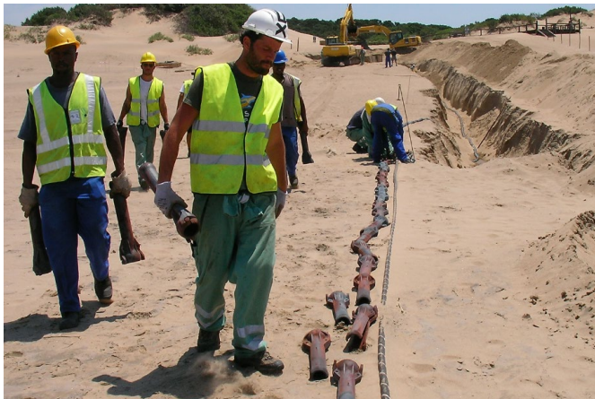
Figure 2-16 Articulated pipe being fitted onto cable example
