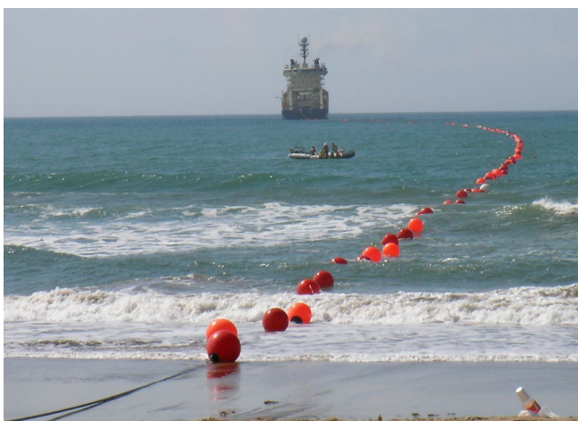
Figure 2-14 Typical shore-end landing utilising flotation buoys
